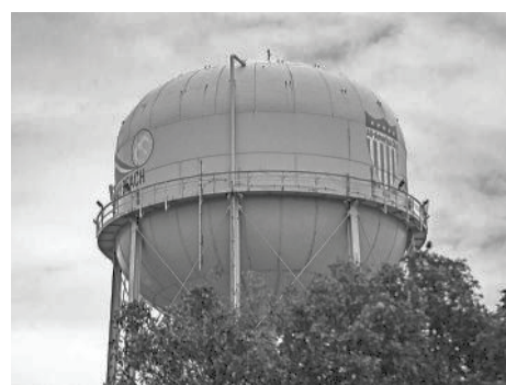
Delray Beach reached a settlement to pay $818,500 to resolve Christine Ferrigan’s whistleblower lawsuit in which she claimed to have been fired for her reports as a wastewater inspector. The city commission approved the deal at a recent meeting. THOMAS CORDY/PALM BEACH POST
